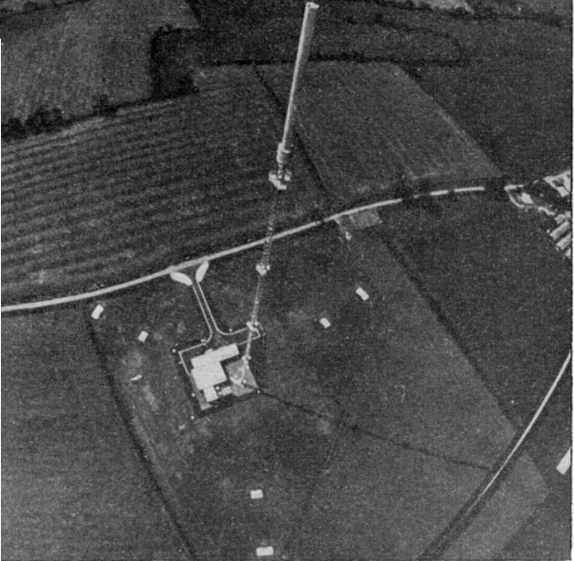
FIGURE 4. A 385 m television mast similar to one at Belmont used to carry meteorological instruments.
